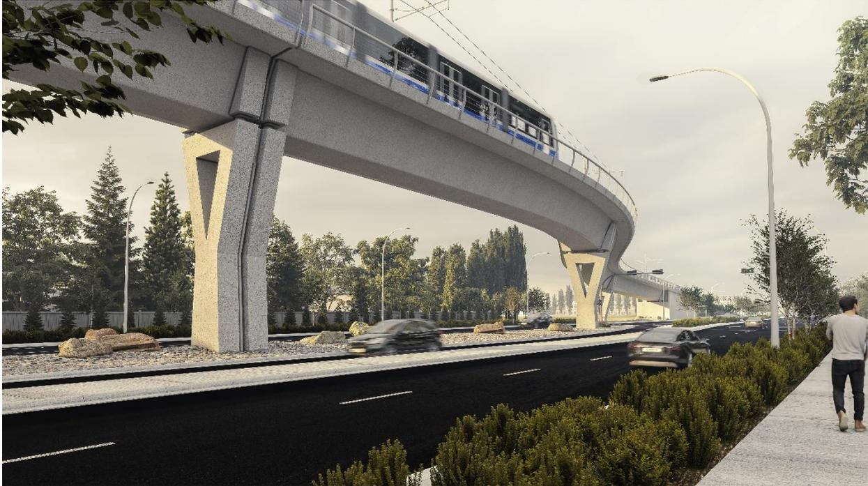
The Valley Line West LRT will feature an elevated guideway that runs along the north side of 87 Avenue between 163 Street and 182 Street. The guideway will feature two new transit stations: Misericordia Station and West Edmonton Mall Station. Marigold Infrastructure Partners (MIP) will begin constructing the guideway by drilling the foundations at 174 Street and working eastward toward 165 Street.
